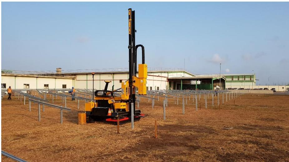
Our standard mould for ground poles is 80x40 C shape.
